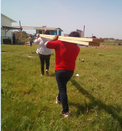
Work on Playa Bagdad Techado
